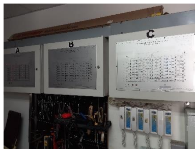
Graphic Annunciator Fire Alarm System
