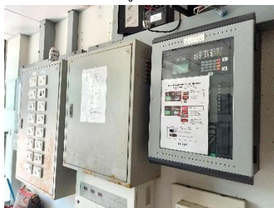
Fire Alarm Control Panel
